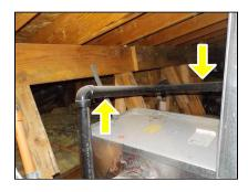
REPLACE (3) There are two or more plumbing vents which insufficient height which should rise six inches above the roof and should be serviced. Evaluation and repair by a licensed Plumber is recommended. (seller's invoice states the flashings were replaced)
