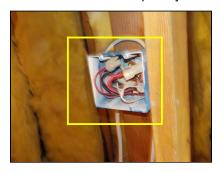
SAFETY CONCERN (2) The electrical wiring in the attic should be evaluated for the following reasons: Exposed single wire, Romex not mounted within 12 inches of a junction box, junction box not mounted to framing, etc. Evaluation and repair by a licensed Electrician is recommended.
