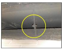
REPAIR / REPLACE (2) The damper-stops are missing at all the chimneys and should be replaced to lock the dampers open for safety. Evaluation and repair by a licensed Chimney Contractor is recommended.
