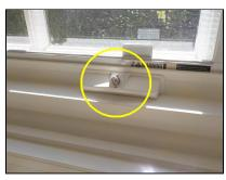
REPLACE (3) A casement window in bathroom 5 has a missing crank mechanism cover which should be replaced. Evaluation and repair by a licensed Window Contractor is recommended.
