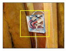
(2) The electrical wiring in the attic should be evaluated for the following reasons: Exposed single wire, Romex not mounted within 12 inches of a junction box, junction box not mounted to framing, etc. Evaluation and repair by a licensed Electrician is recommended.
