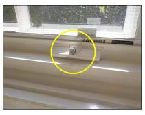
(3) A casement window in bathroom 5 has a missing crank mechanism cover which should be replaced. Evaluation and repair by a licensed Window Contractor is recommended.
