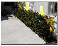
EXPLORE FURTHER (3) There is grass plated against the back foundation stem wall which should be maintained two feet away to avoid damage or moisture intrusion. Evaluation and repair by a licensed Landscape Contractor is recommended.
