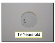
EXPLORE FURTHER (2) There is an alarm dependant smoke detector that is beyond the scope of a home inspection and should be demonstrated to be functional by the Security Company Contractor.
