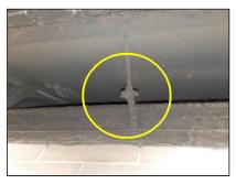
(2) The damper-stops are missing at all the chimneys and should be replaced to lock the dampers open for safety. Evaluation and repair by a licensed Chimney Contractor is recommended.
