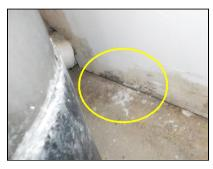
REPAIR / REPLACE (2) There is mineral encrustation on the fittings as a consequence of leaks. Evaluation and repair by a licensed Plumber is recommended. (dry when inspected)
