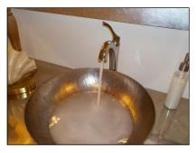
(2) The right mechanical sink stopper in bathroom 5 will need to be serviced to function properly. Evaluation and repair by a licensed Plumber is recommended.
