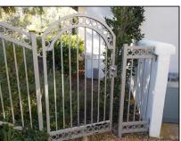
SAFETY UPGRADE (2) Installing audible alarms and self closing hinges on doors that give access to the pool and spa are recommended for safety if children occupy or visit the property. Evaluation and repair by a licensed Contractor is recommended
